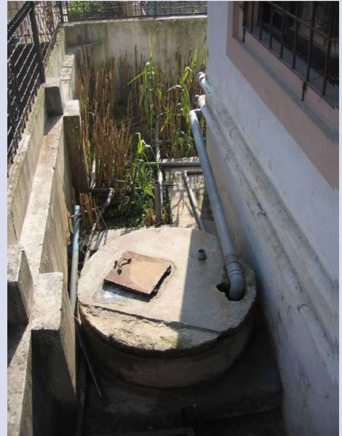
Dug well for groundwater collection and recharge
