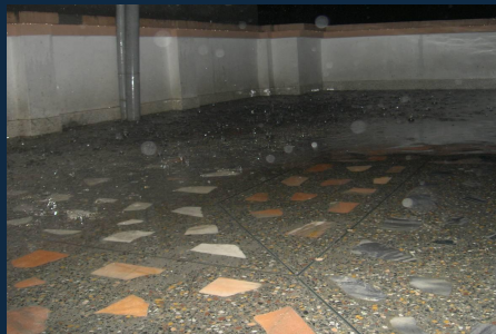
Roof as Rainwater Catchment
