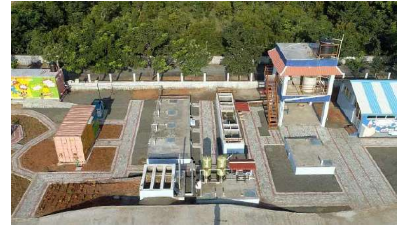
FSTP at Periyanaicken-Palayam (PNP)
