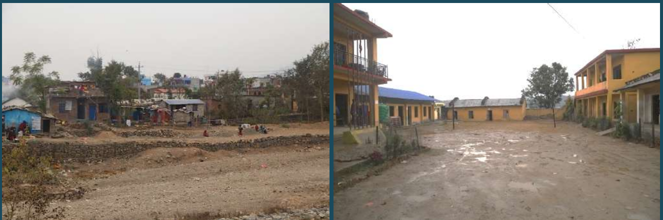
Water sensitive settlements along seasonal water streams (left) Schools located in flood prone area (right)
