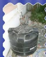
Rainwater first flush tank to washout dirt
