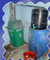
Urine & faeces collection tanks at the basement
