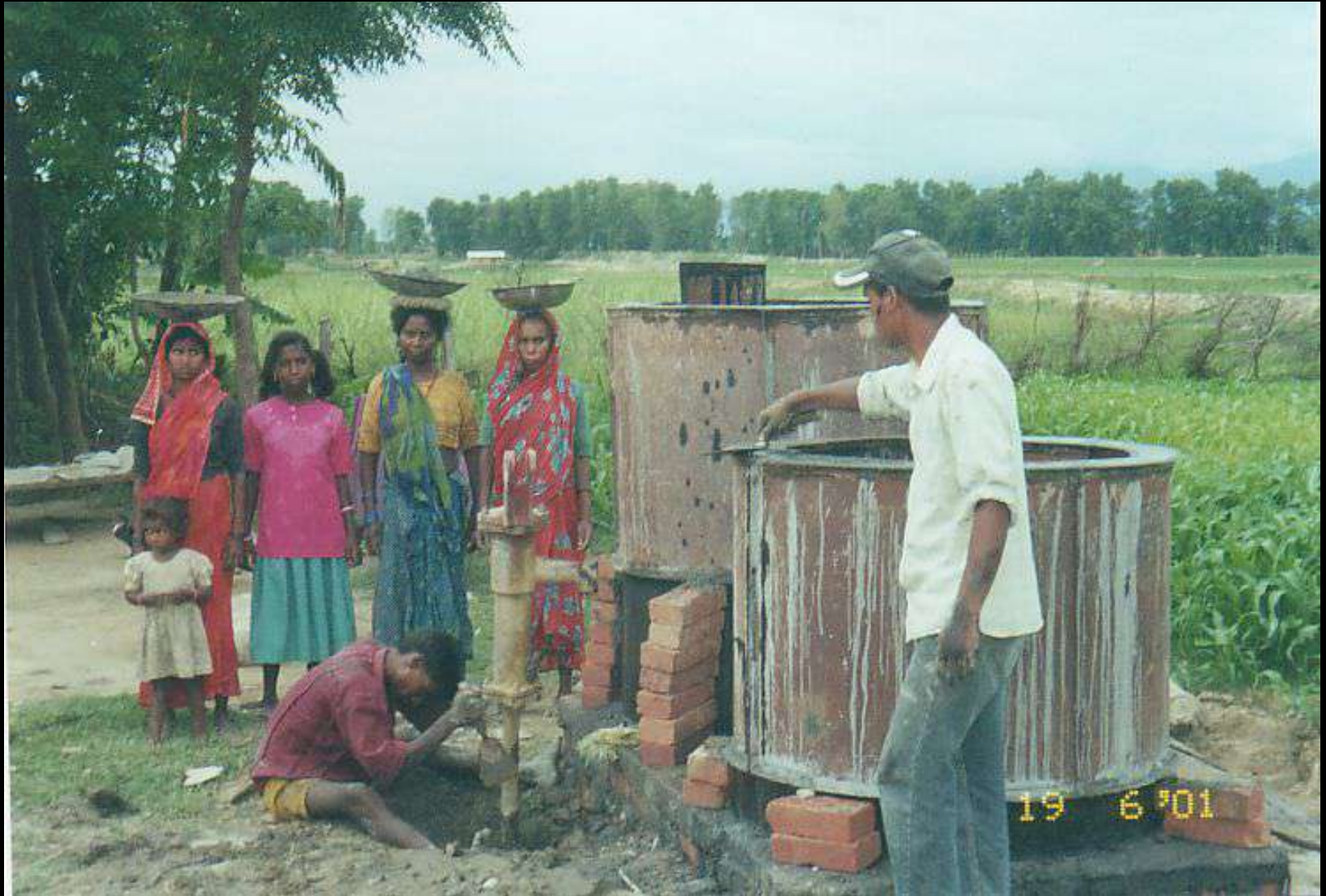
Community level Arsenic Removal Treatment Plant under construction ( Nawalparasi)
